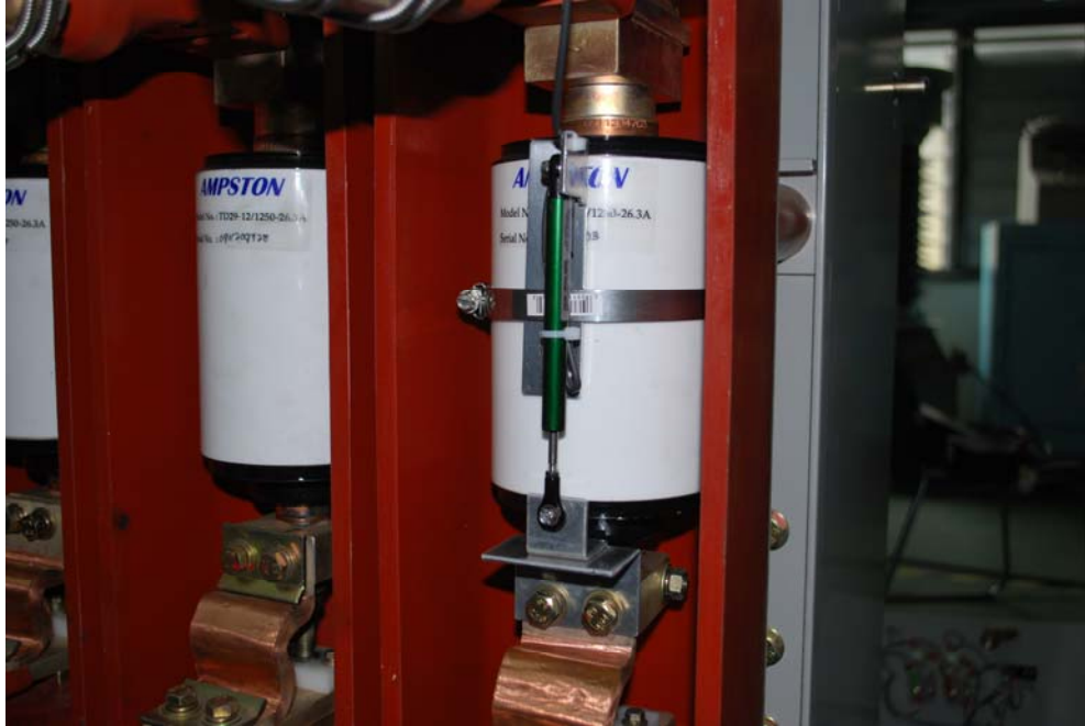
Resistor Transducer on Vacuum Circuit Breaker
